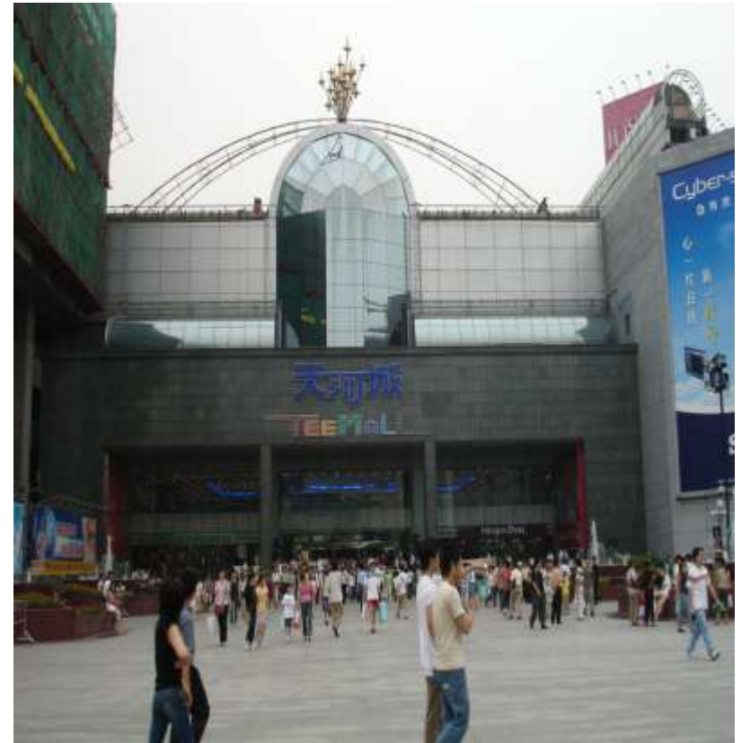
A new mall in Guangzhou in 2006
